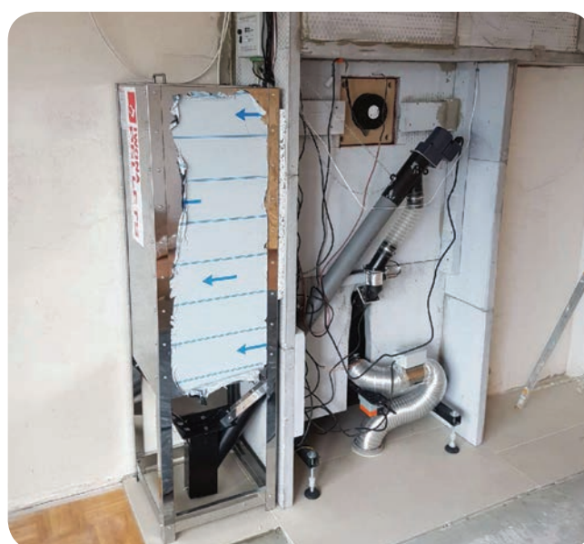
Exemplary installation with a tank in the room behind the fireplace
