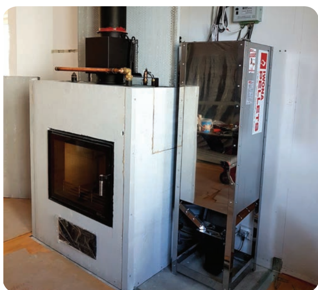
Exemplary installation with a tank beside the fireplace
